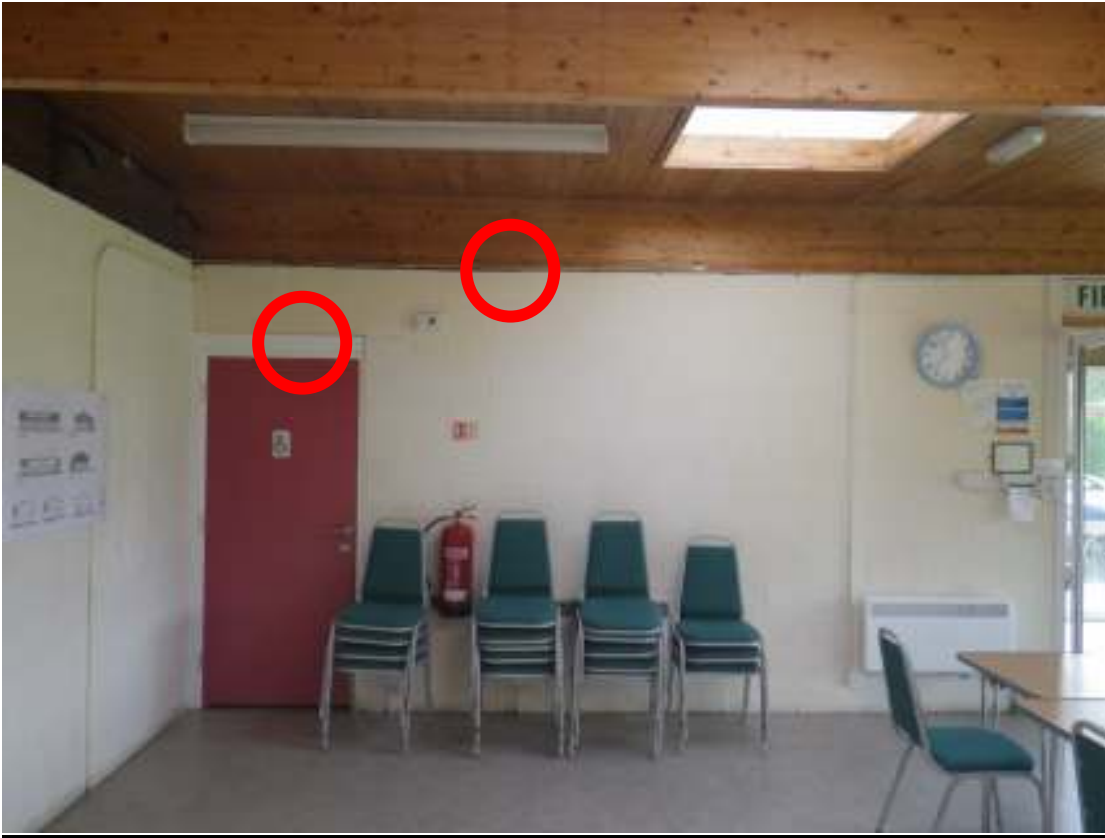
View towards disabled person toilets
