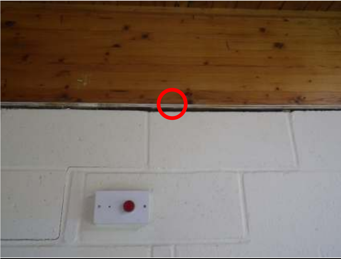
Opening up under the timber glulam beams due to the concrete slab settling
