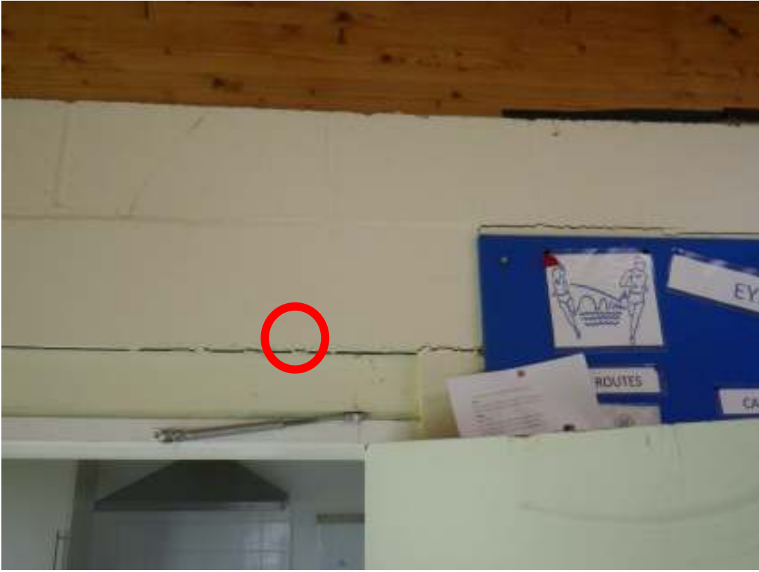
Cracking above the doorways
