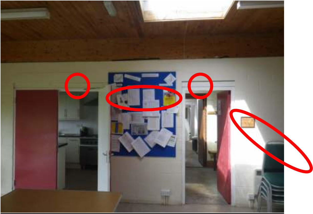
Cracking above the doorways
