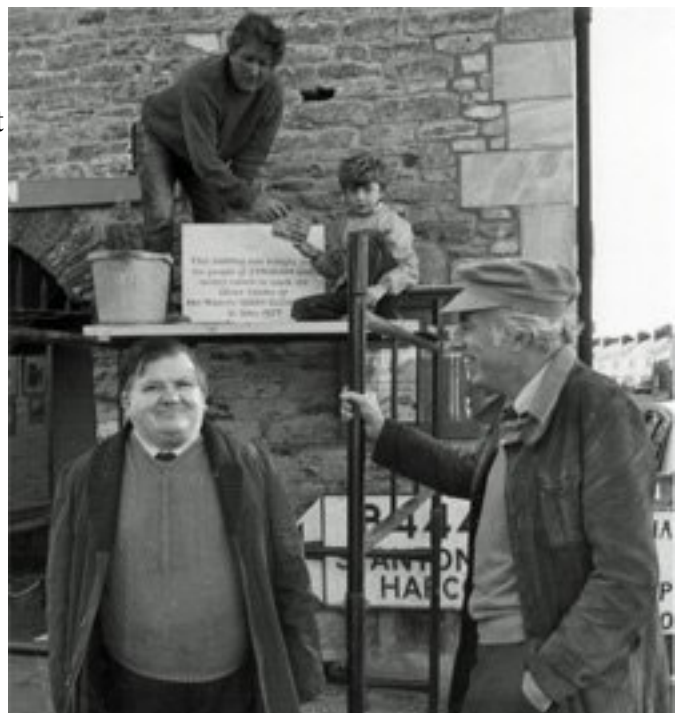
David Wastie and Don Chapman at installation of a memorial plaque on the Bartholomew Room; image © Sue Chapman, 1982
