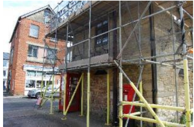
Photograph 4. Photograph showing the eastern elevation of the building.
