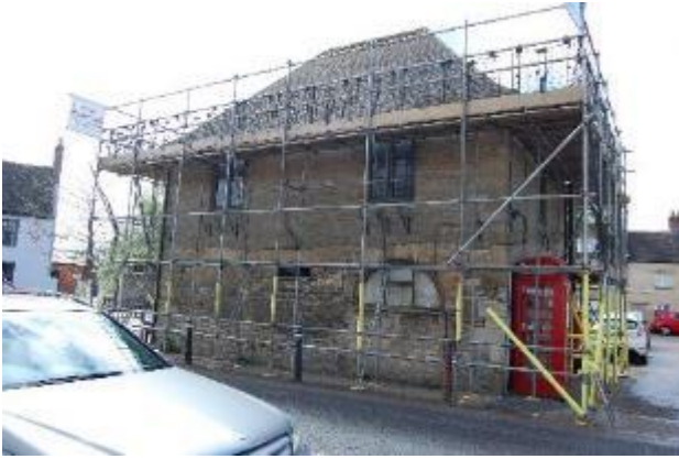
Photograph 1. The northern elevation of the Bartholomew Building.
