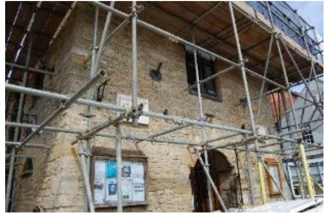
Photograph 2. Photograph showing eastern elevation of the building.
